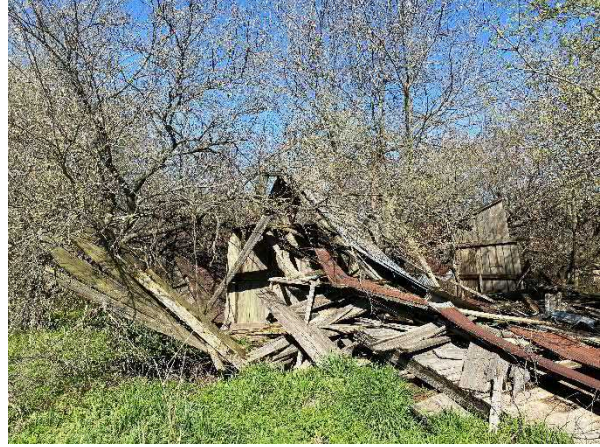
Photo 14 View of former shed debris on the west-central portion of the site.
