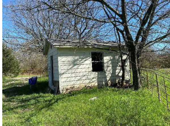
Photo 10 View of the shed near the house.
