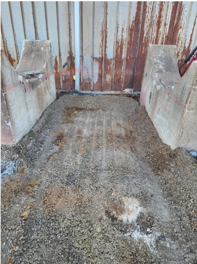
Tank Soil area Post remediation Fill dirt added post remedial
