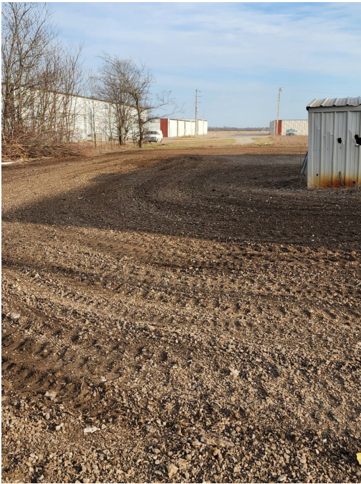
Post remedial Action Tilling and Dragging
