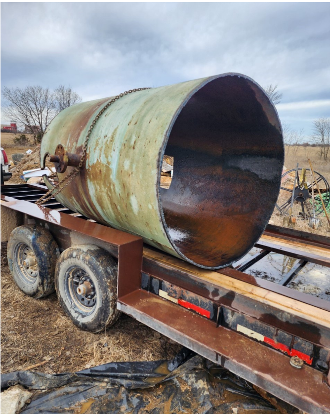
Cut up of tank after decontamination inside and outside surfaces
