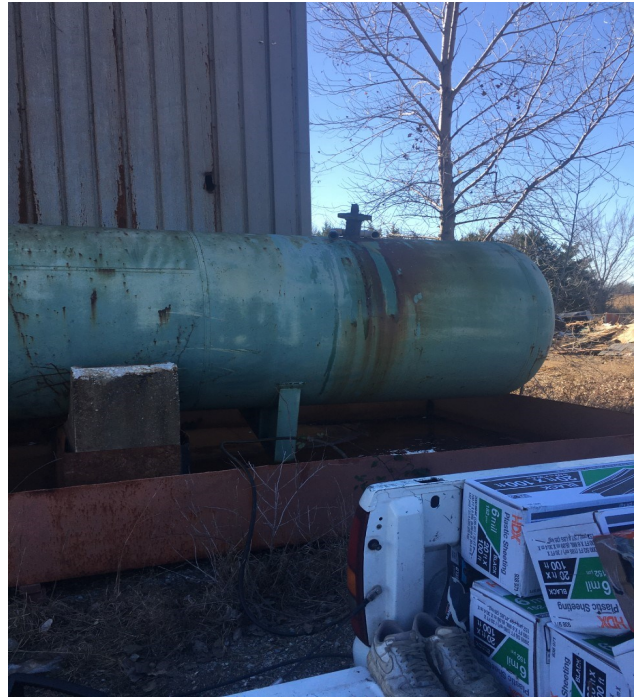
Lowered end of Tank with retain #2
