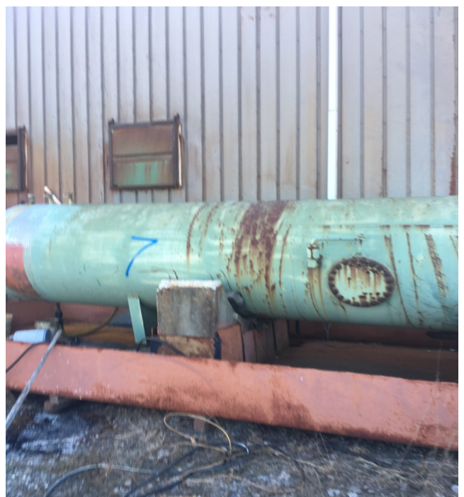
Mid Section of Storage Tank Pre remedial Activity #4
