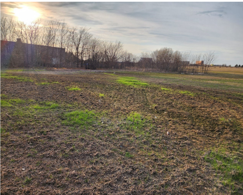
Seeding activity post remedial activity for erosion control
